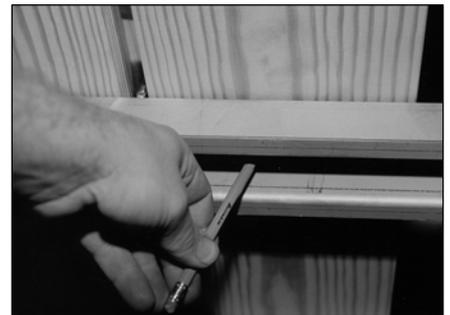
20. The rear cross sill also receives a bed-to-frame bolt. Mark the boards through the rear cross sill brackets.
