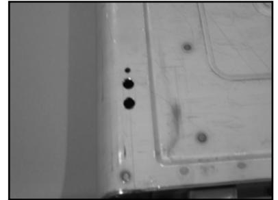
5. Using a small high speed cutting wheel, connect the two 3/8" diameter holes by cutting the metal out between them. This will create the slot that the knob on the latch will slide in.
