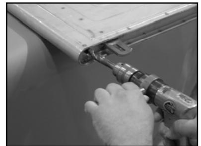
8. Slide the latch sleeve into the tailgate through the 5/8" hole until the small threaded hole lines up with the small hole in the tailgate. Thread the 10-32 button-head screw through the tailgate into the latch sleeve and tighten with the supplied 1/8" hex wrench. Check the alignment of the slot in the tailgate with the slot in the latch sleeve.
